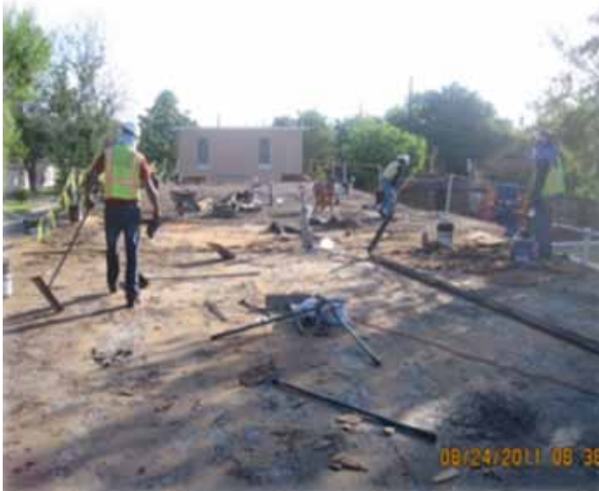
Scraping and removing the old roof system Buena Vida Housing Development
